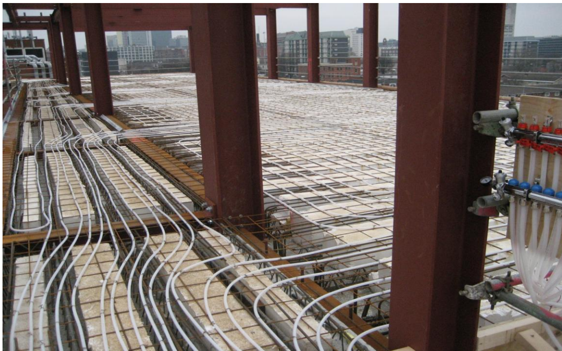
Installation of under floor heating
